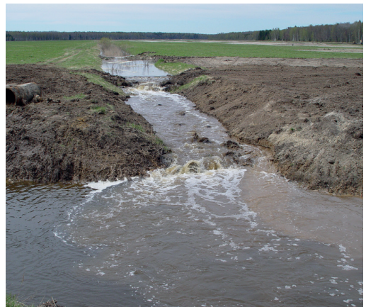
Fig. 21.6.8. A weir on the River Slampe to raise the water level. Photo: G. Pāvils.
